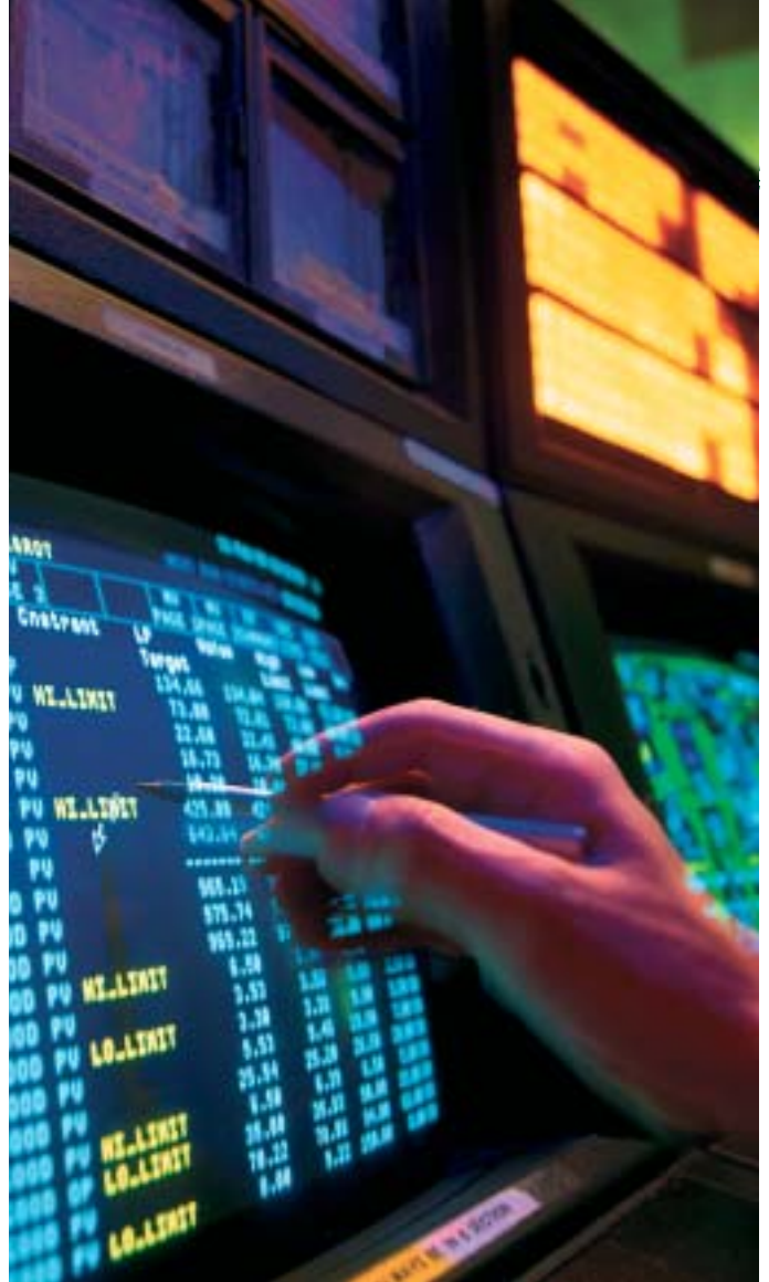
In a centralised remote monitoring facility, specialists can be employed to provide support to a far greater number of plants simultaneously.
